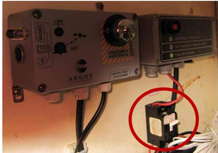
**Figure 29:** Argos junction box with on/off switch.
