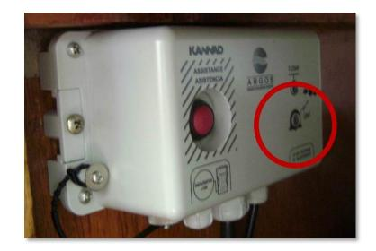
Figure 30: Argos junction box switched off.
