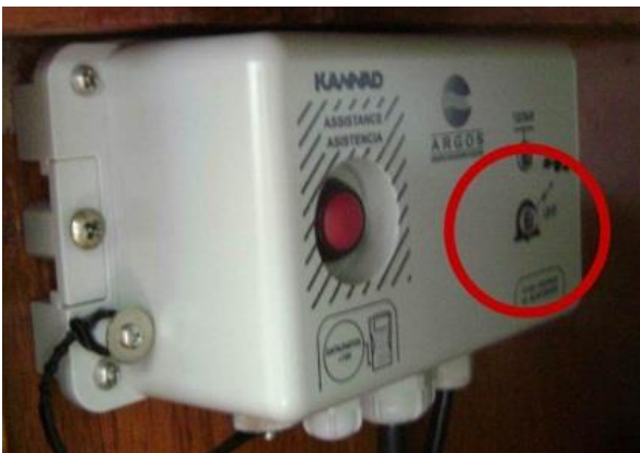
Argos junction box switched off.
