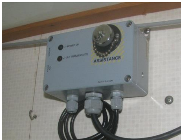
Figure 26: Junction box for the Argos MAR G E unit and Junction box of a MARGE V2 unit.
