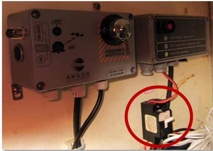
Figure 29: Argos junction box with on/off switch.
