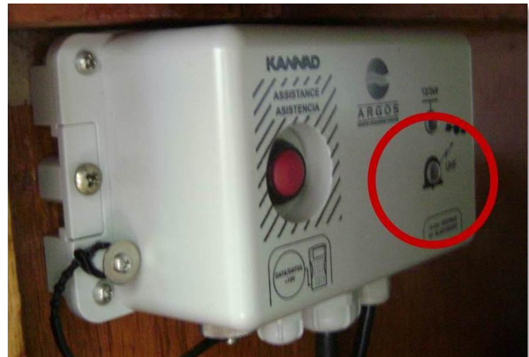
Figure 30: Argos junction box switched off.
