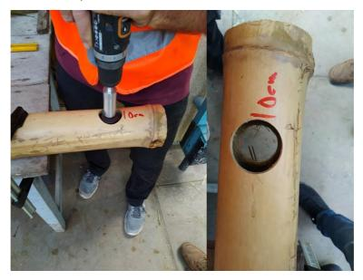
4. Drill a whole of about 20mm diameter through the bamboo cane on both sides (for the rope)
