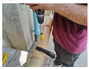
5. Interlock bamboo canes to form a cross joint to ensure holes have been made to specifications
